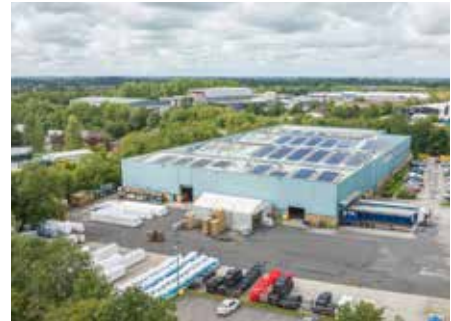
Manufacturing plant, Preston, UK
